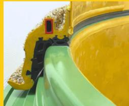
FULLY LINED MANHOLE INCLUDING JOINT LINING
